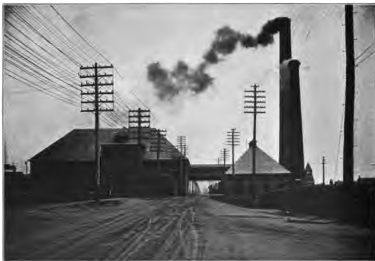
CALUMET & HECLA—"SUPERIOR" POWER PLANT. (Photo by Nara, Calumet.)
